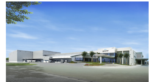
Location expansion project in Thailand
