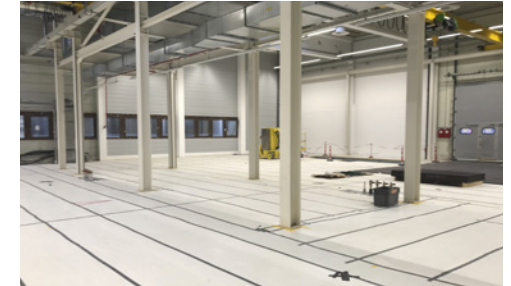
Infrastructure project at the Frickenhausen site, Germany
